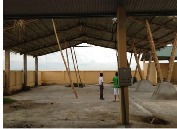
In Vietnam a composting facility processing around 800 t/y of palletised compost based organic fertiliser has been implemented. A bamboo hangar has been designed and constructed developing a particular technological detail to maximise the span of the trusses using relatively short bamboo canes. In the framework of the project 150 biogas fix dome have been delivered.
